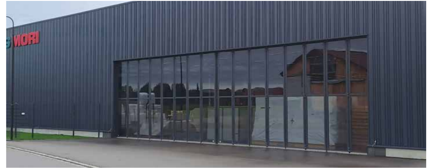
Schiebefalttor Deckel Maho 17,5 m x 5m Sliding folding door Deckel Maho 17,5 m x 5m
